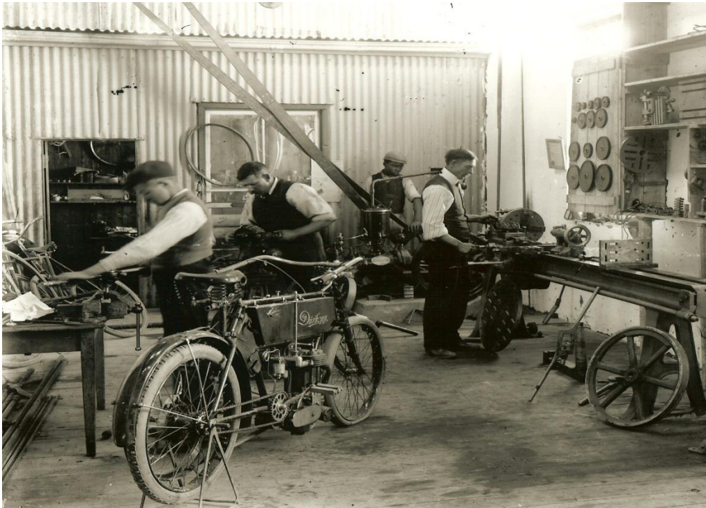
1911 DURKOPP IN WORKSHOP FOR REPAIRS
